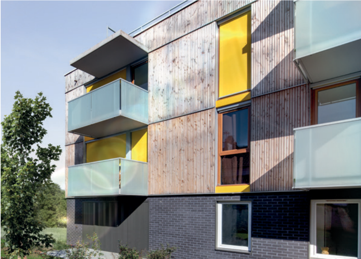
Installation with visible cover panels
